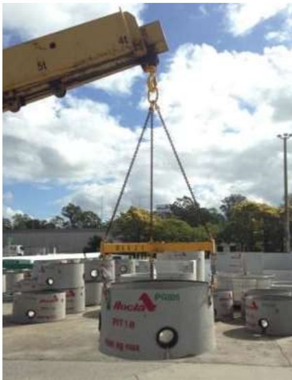
Fig 1.1 – Use of lifting spreader beam
