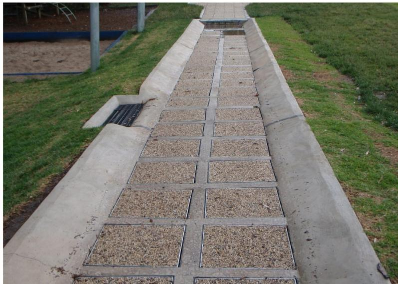
**Figure 2:** The stormwater treatment system at Syndal South Primary School.
