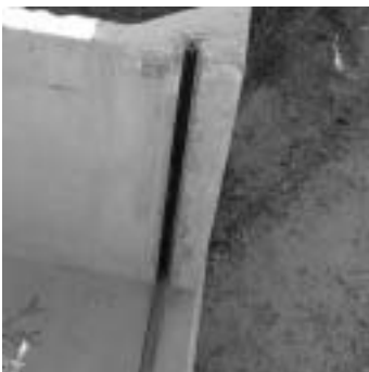
L-Stop with rubber insert for slide
