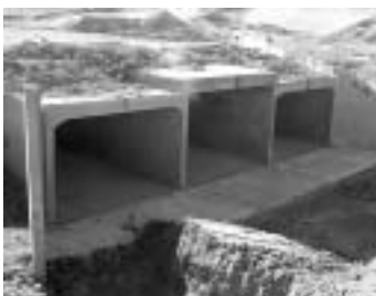
Large multi-cell box culvert headwalls
