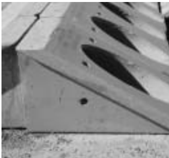
Low-profile sloping face headwall
