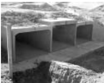
Large multi-cell box culvert headwalls
