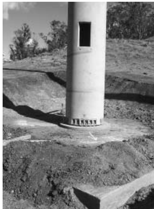
Concrete pad footing for installation on rock
