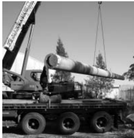
Unloading poles with chain sling
