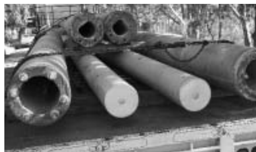
Poles of different diameters require support bearers and timber packing
