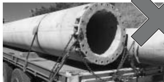
Poles or piles must not be secured via joint lugs
