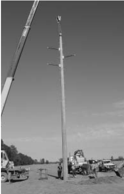
Placing the pole
