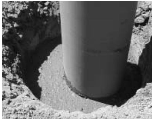
Backfilling with concrete
