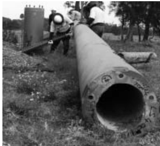
Installing fittings before erection
