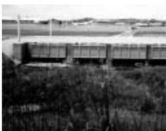
Box Culvert Floodgates
