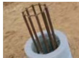
PREFABRICATED STEEL REINFORCEMENT CAGE FOR HEADSTOCK CONNECTION
