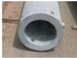
INTERNAL SCABBLING OF PILE
