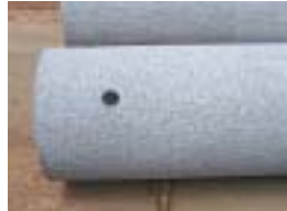
EXTERNAL SCABBLING OF PILE
