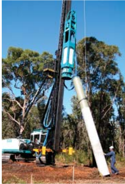
DURASPUN® CONCRETE PILE BEING DRIVEN WITH HYDRAULIC DROP HAMMER.
