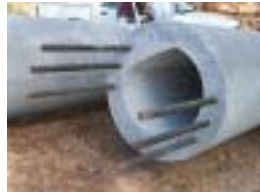
HEADBARS EMBEDDED IN PILE
