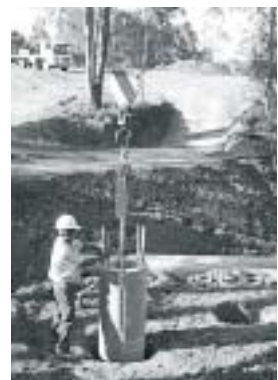
DURASPUN® CONCRETE PILE BEING POTTED INTO PRE-DRILLED HOLE.
