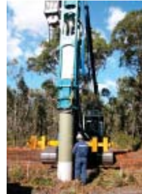
DURASPUN® CONCRETE PILE BEING DRIVEN WITH HYDRAULIC DROP HAMMER.
