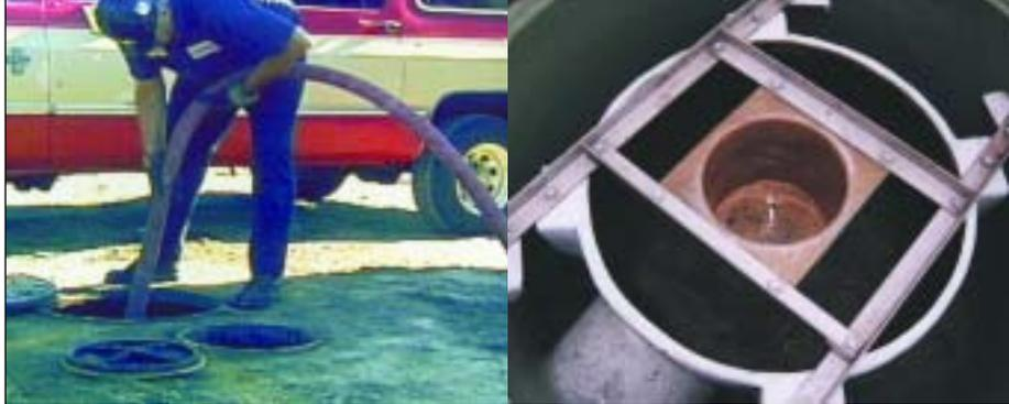
Downstream Defender\* oil and sediment separator captures settleable solids, floatables, oils and grease from stormwater runoff. **Created by Hydro International it is available from Rocla under exclusive license in Australia.**
