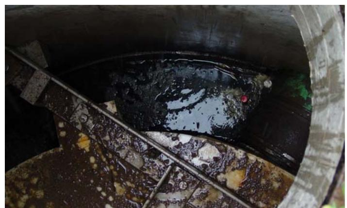
**Figure 7:** View of outer annulus of floatables and oil collection zone
