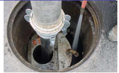
**Figure 5** – Vacuuming Sediment Sump
