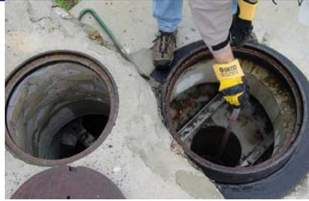
**Figure 4** – Checking Sediment using a Probe
