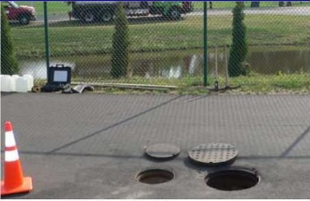
**Figure 3** – Inspection and Maintenance Covers
