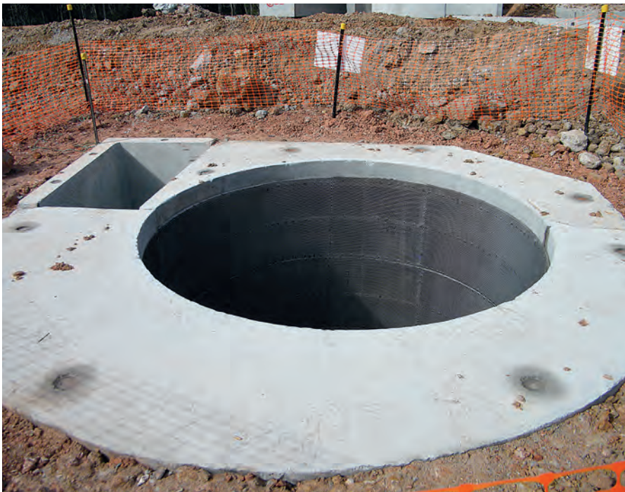
In North Lakes, the largest gross pollutant trap installed by Rocla in Queensland had a footprint of 7m by 5m and was designed with the assistance of SWATT modelling software.
