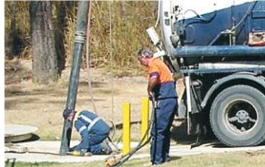
Suction cleaning is used for most proprietary GPT's. Even if a more cost effective method is used at shorter intervals, suction cleaning is recommended for CDS® Units at one to two year intervals so that a thorough inspection of the screen and lower chambers can be carried out. Physical entry may or may not be required.
