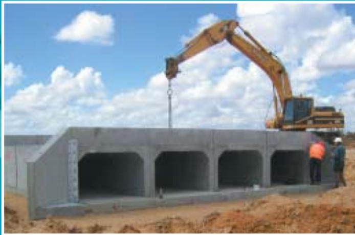
Rocla® reinforced concrete box culverts (RCBCs) are the fast, easy solution for applications under roads, railways and runways as drainage culverts, underpasses or service ducts. Precast units mean fast installation with minimal disruption to services and traffic.
